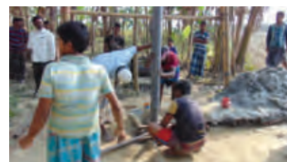
Photo: Installing Irrigation DTW in Ganna village
