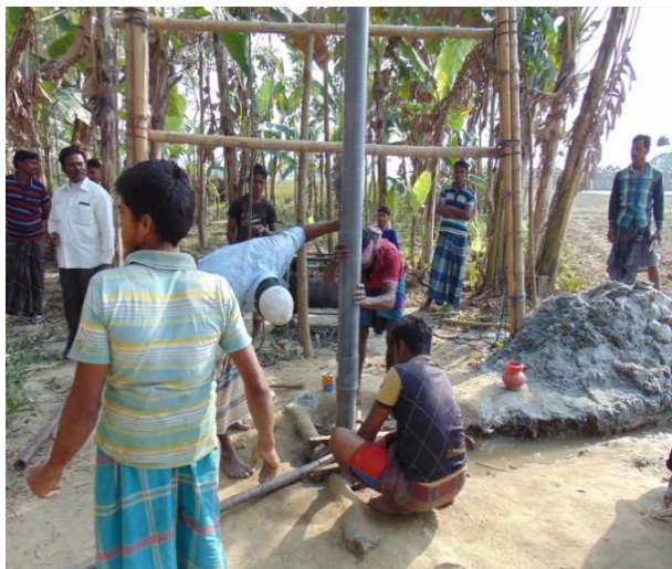
Photo 6: Installing Irrigation DTW in Ganna village
